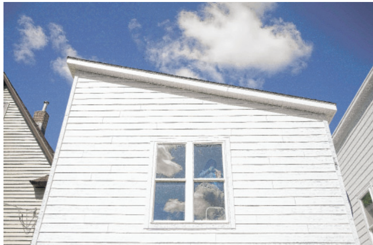
Volunteer Yolanda Perry paints the inside of a house. Habitat for Humanity Chicago and the Cook County Land Bank Authority, in partnership with By The Hand Club, are building three single-family homes in Austin that will be owned by Austin residents.
